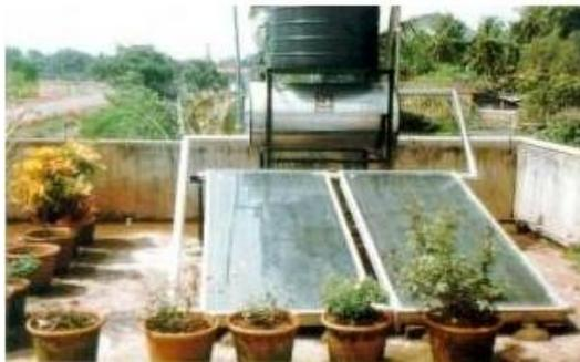
Fig: 4 Solar water heating system (SWH)
