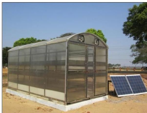
**Fig. 1 Forced ventilated solar green house dryer**
