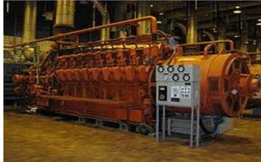
Fig:-Big Diesel Generator Used For Backup Power
