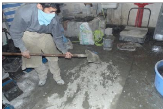
Figure 1.4 – Preparation of concrete mix with bacteria
