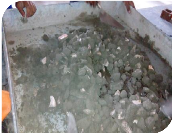
Figure: 8 Mixing of Concrete
